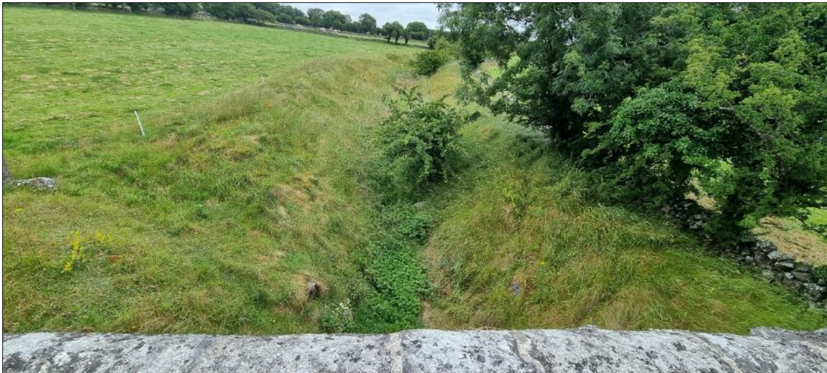
Plate 4.2 Representative image of site A2 on the Glennafosha River at Claretuam Bridge, July 2022 (ephemeral, dry channel)
