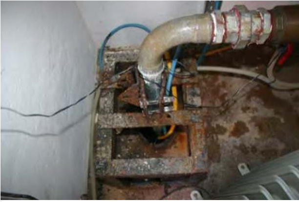
Photo 1: Borehole headworks
