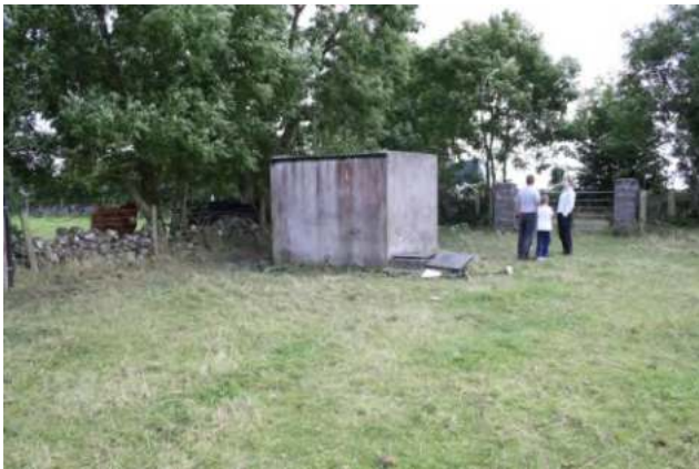
Photo 1: Pumphouse and adjacent borehole at ground level to right of pumphouse
