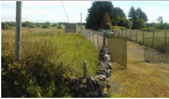
Photo 1: Anbally & District GWS view south across GWS compound
