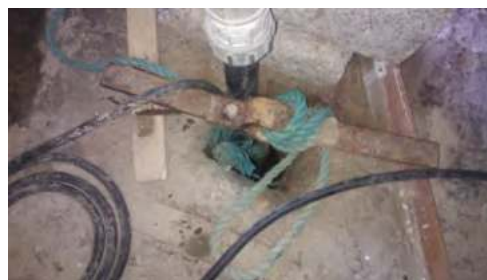
Photo 4: Old hand pump borehole inside pumphouse
