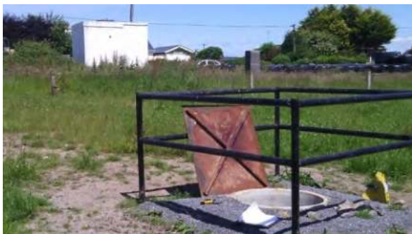
Photo 1: Rusheens GWS wellhead with pump house to rear (view northeast)
