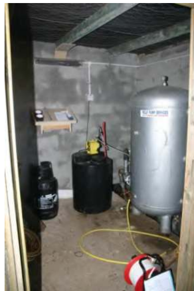
Photo 4: Inside view of pumphouse
