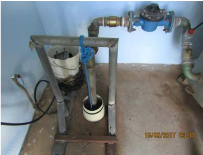
Photo 2 Cluide - Cahermorris GWS borehole
