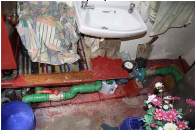
Photo 3: Flowmeter on mains line
