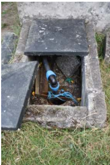
Photo 3: Borehole chamber
