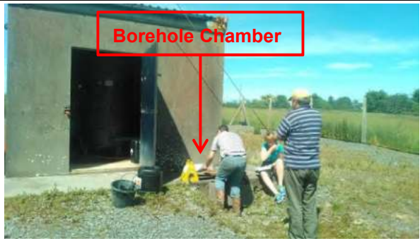
Photo 2: Anbally & District GWS – Pump house and adjacent well chamber (view NE)
