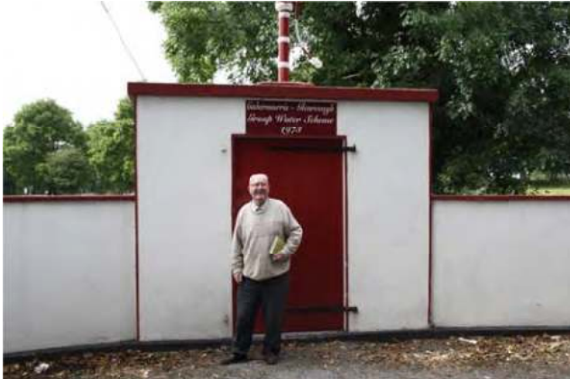
Photo 1: Pumphouse. Borehole head located within pumphouse
