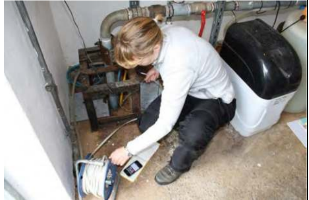
Photo 2: Borehole headworks (note split galvanised sheet cover)
