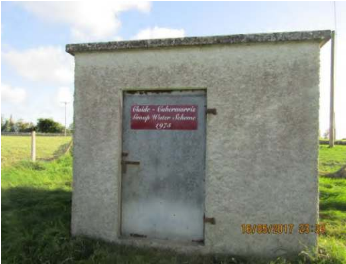
Photo 1 Cluide - Cahermorris GWS borehole pump house
