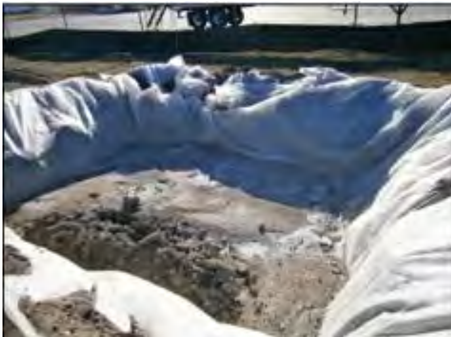
Plate 4-4 Concrete Washout Area
