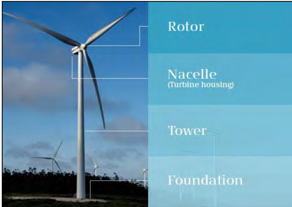
Plate 4-1 Wind turbine components
