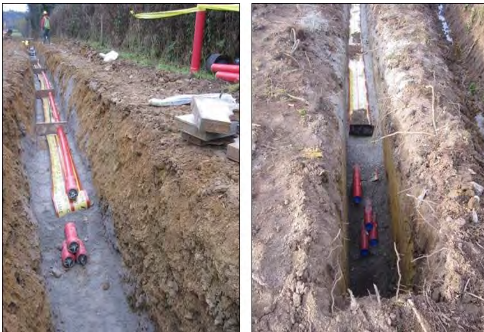
Plate 4-6 Typical Cable Trench View
