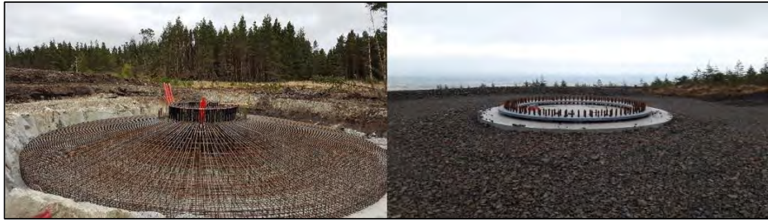
Plate 4-2 Turbine 'Anchor Cage' and finished turbine base
