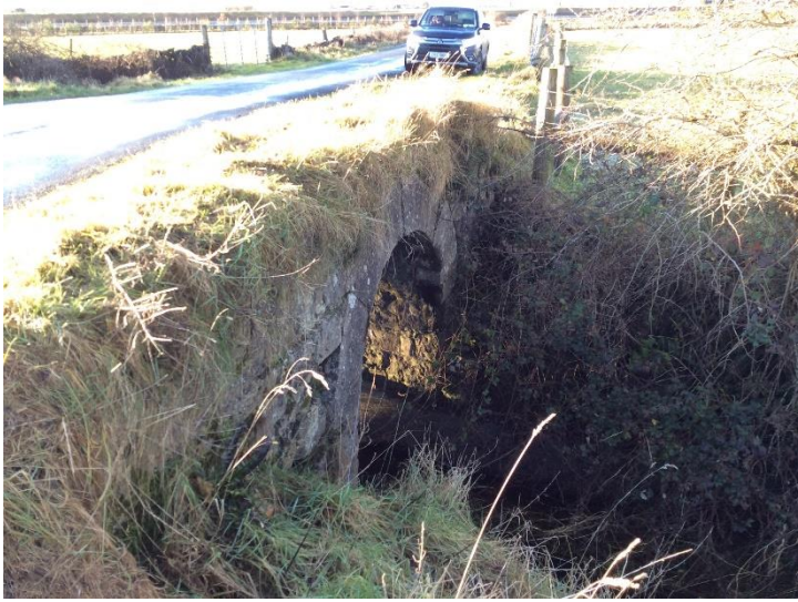
Plate 26: CH3 bridge on proposed underground cabling route.
