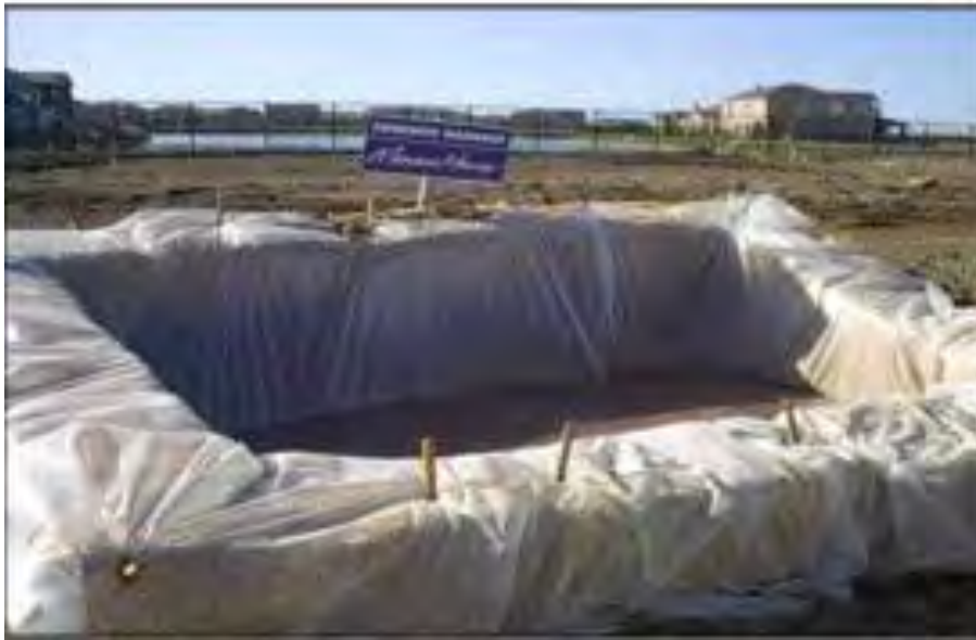
Plate 4-3 Concrete Washout Area
