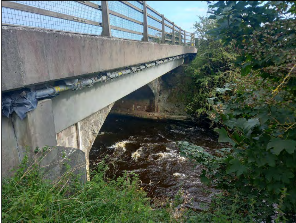
Plate 6-19 Water Crossing 2 over the Clare River
